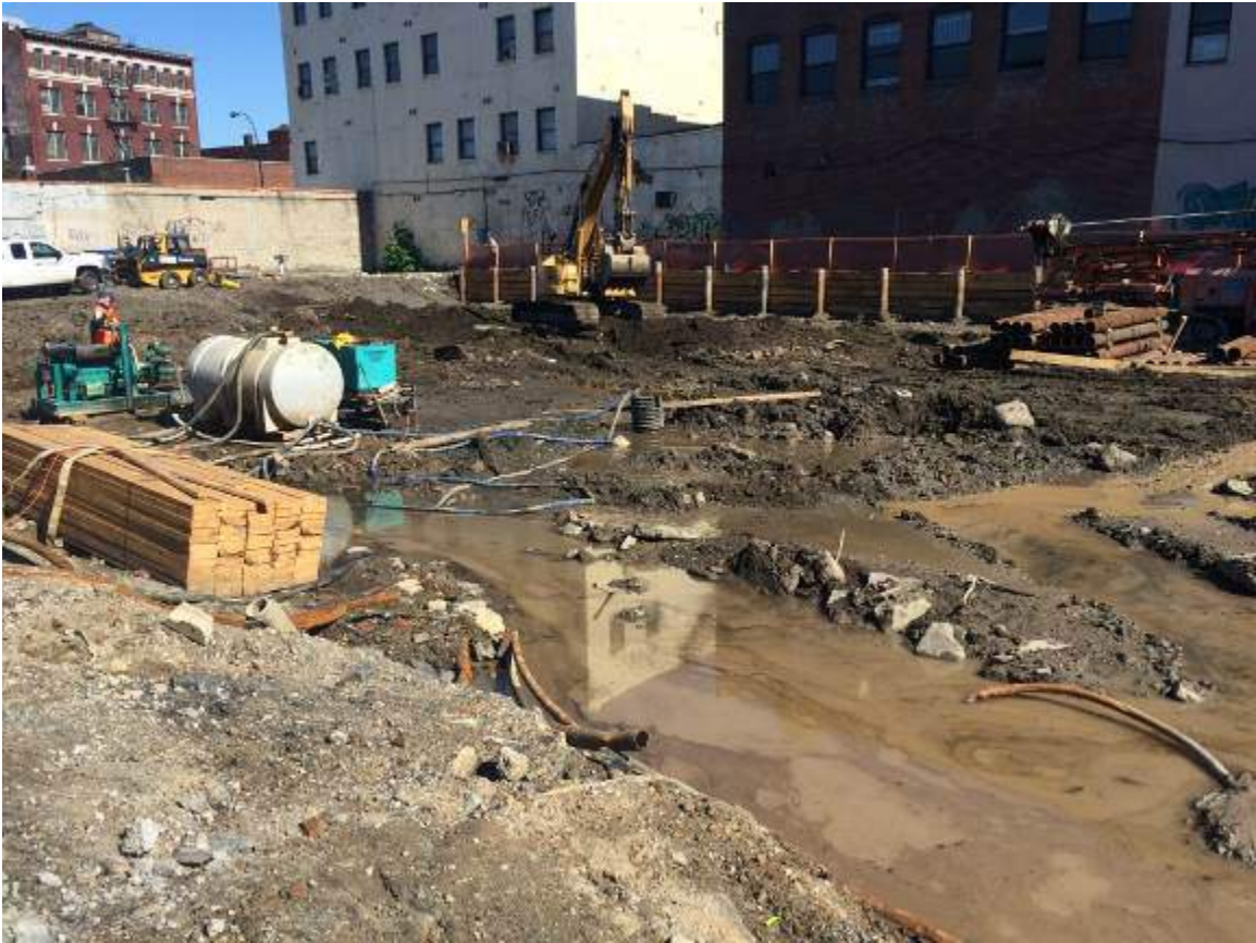
Photograph 23: View of the Site excavation progression, facing north.
