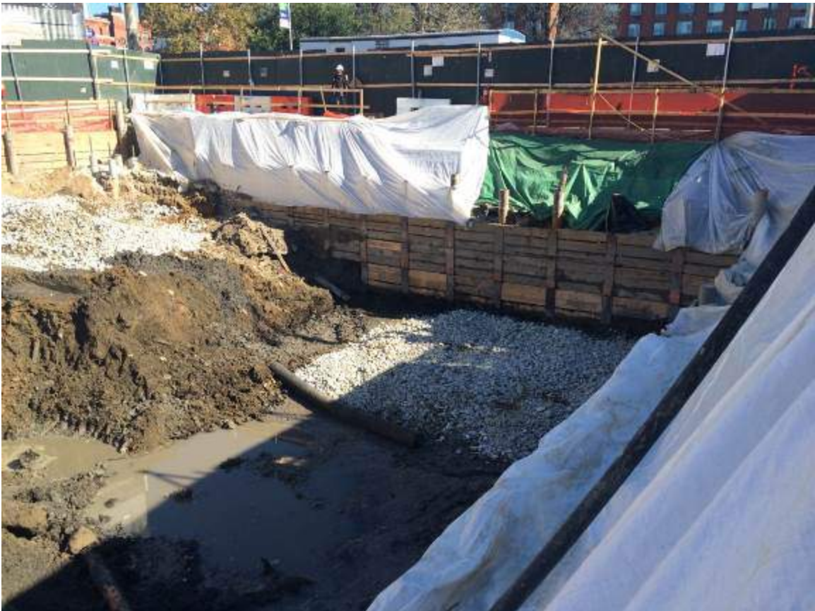
Photograph 34: View of the stone applied on top of the base of excavation area in the southeast portion of the site, facing northeast.
