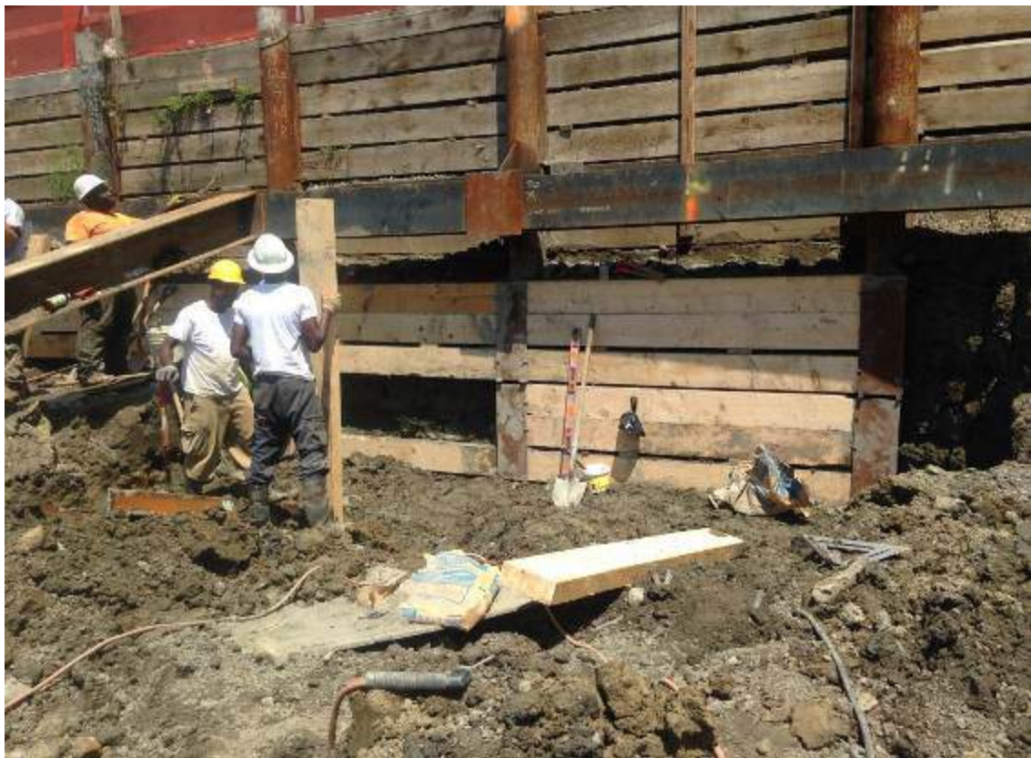
Photograph 72: View of the lagging installation along the northern boundary of the Site, facing north.
