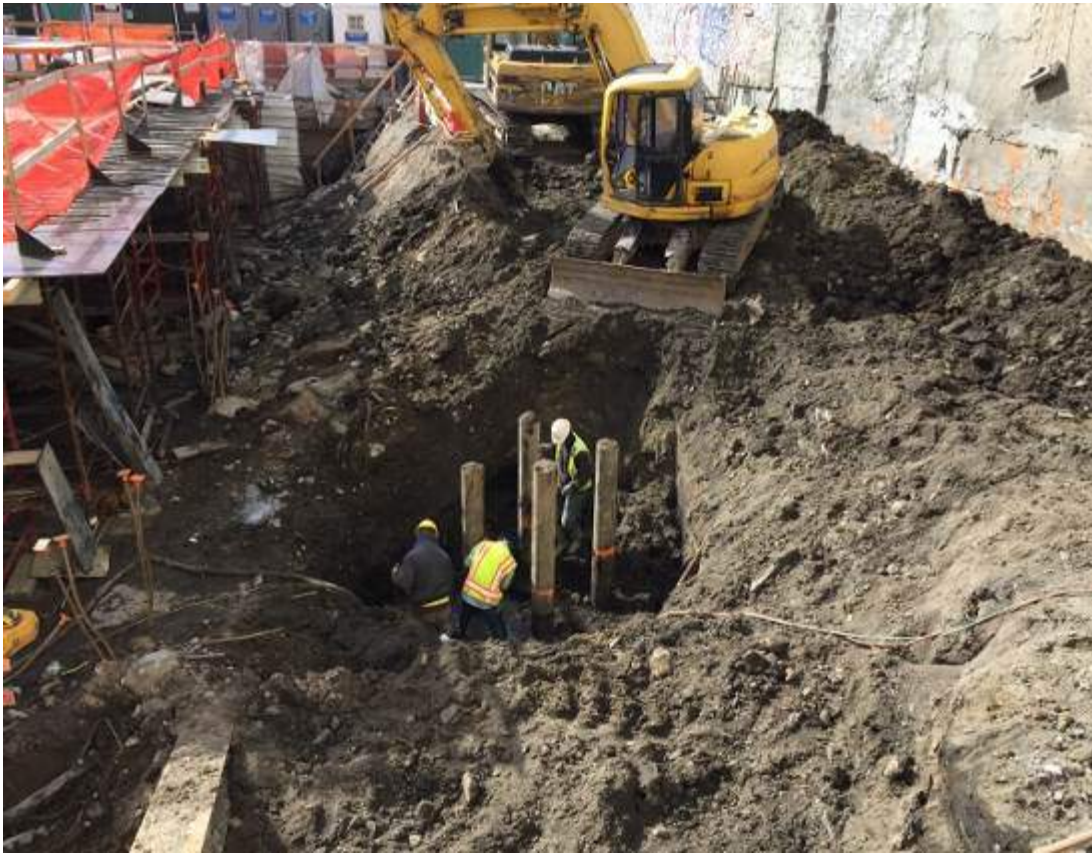
Photograph 101: View of the contractor welding the piles, facing southwest.
