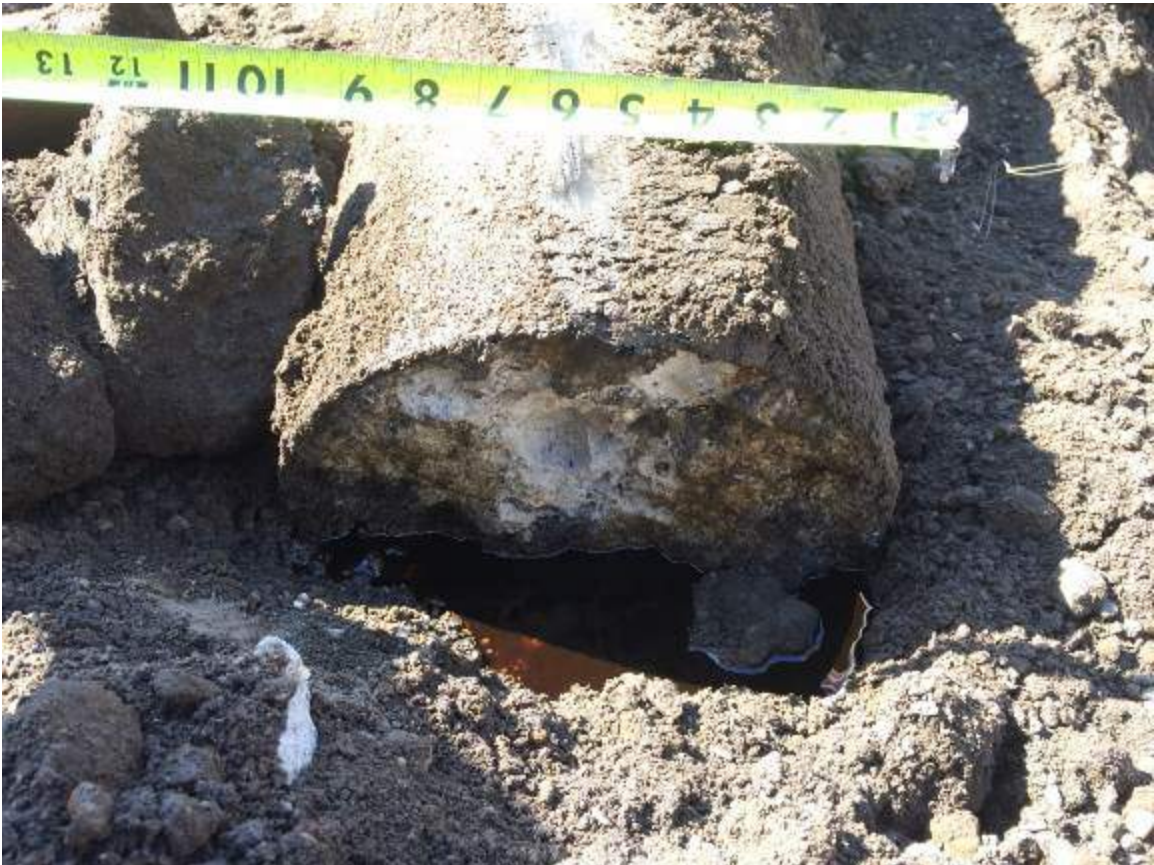
Photograph 26: View of the bottom of Lift-1.
