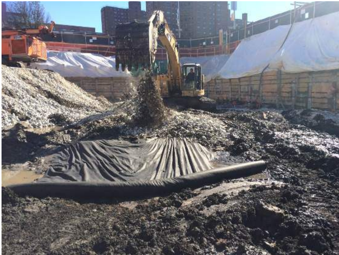
Photograph 36: View of the stone application on top of the base of excavation area facing south.
