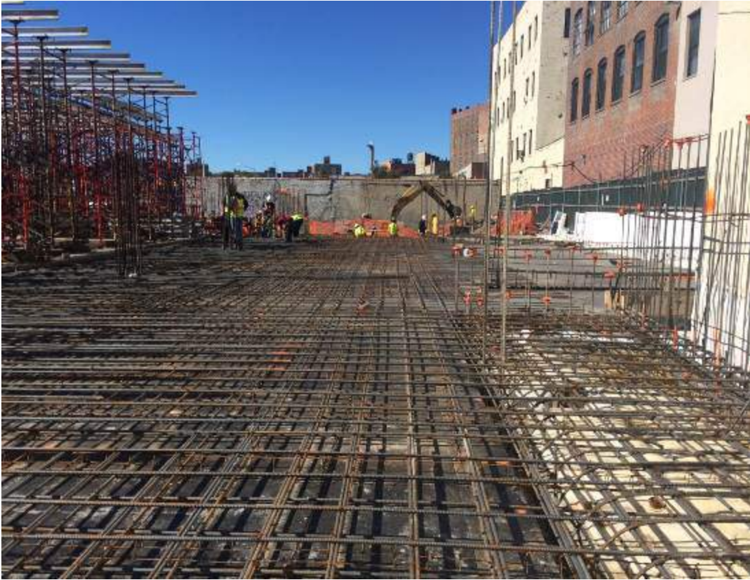
Photograph 91: View of the installed rebar, facing northwest.
