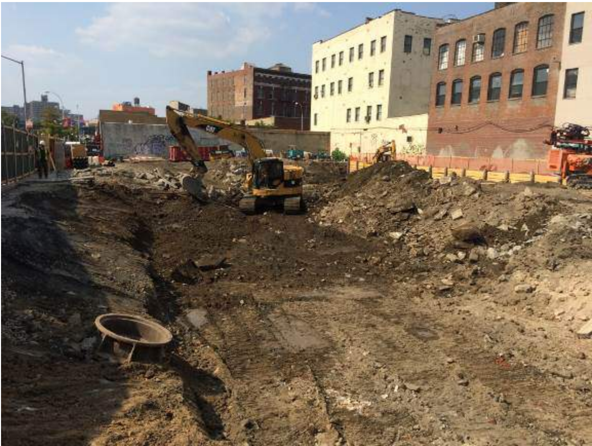
Photograph 17: View of the excavation area progression, facing north.
