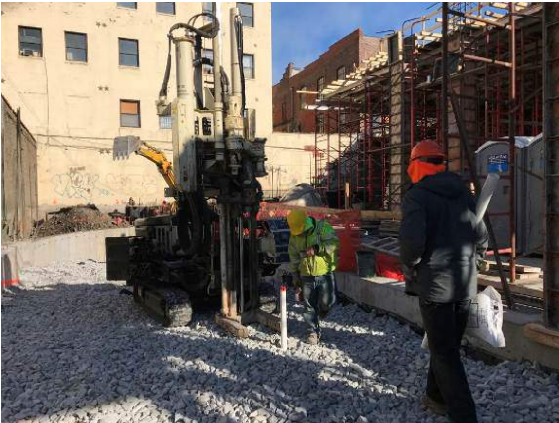
Photograph 127: View of the installed permanent monitoring well (SMW-2), facing northeast.
