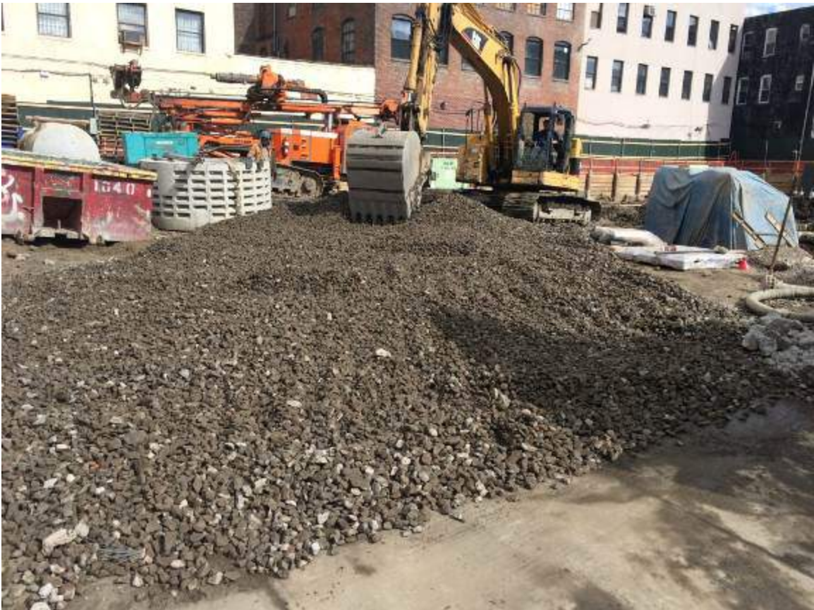
Photograph 32: View of the stone being applied to the Site entrance.
