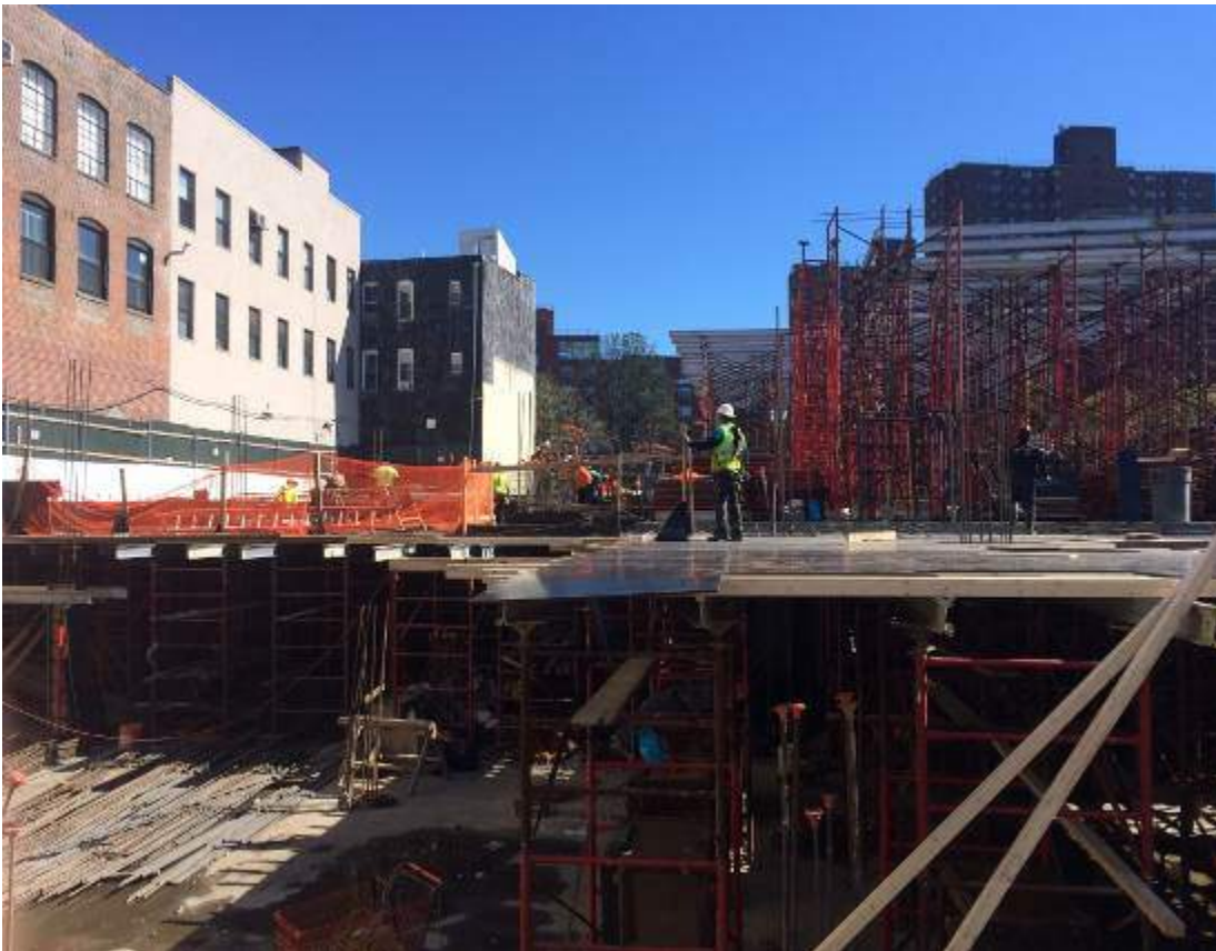
Photograph 92: View of the superstructure installation, facing east.
