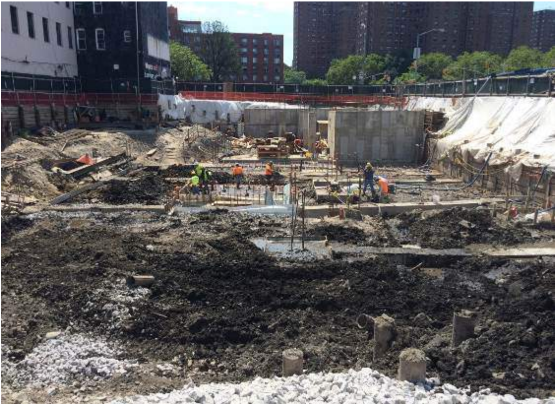
Photograph 61: View of the Site, facing southeast.
