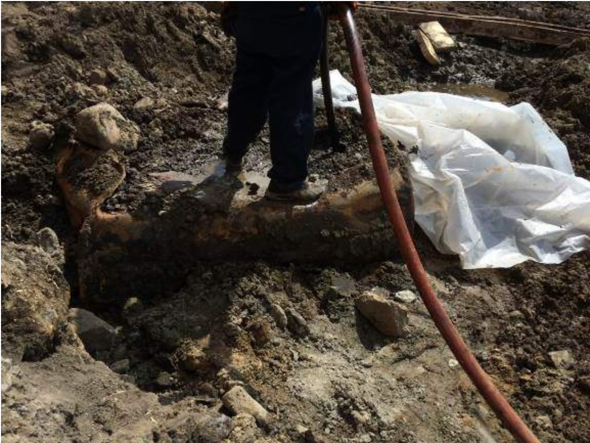
Photograph 21: View of Mercury Tank Cleaners removing the liquid contents from UST-17.
