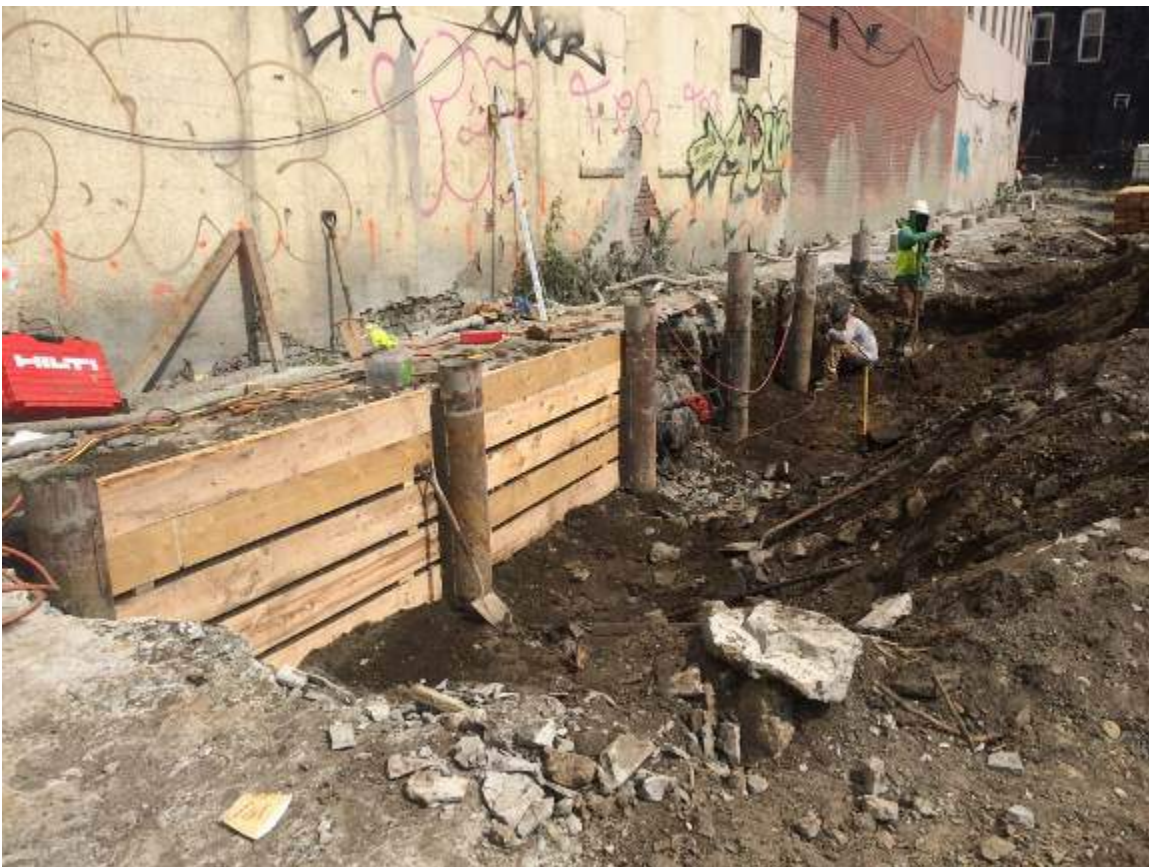
Photograph 4: View of the lagging installation along the northern boundary, facing east.
