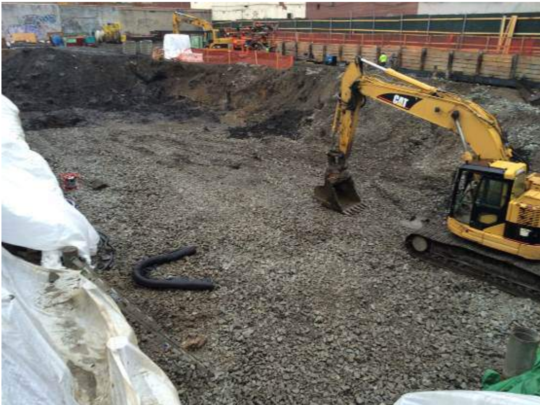
Photograph 38: View of the Site, facing north.
