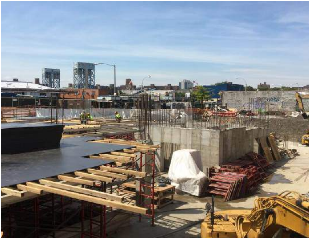
Photograph 82: View of the contractor continuing work on the superstructure, facing west.
