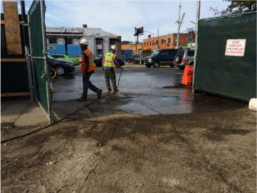
Photo 5 – View of the contractor applying water to the Site entrance.
