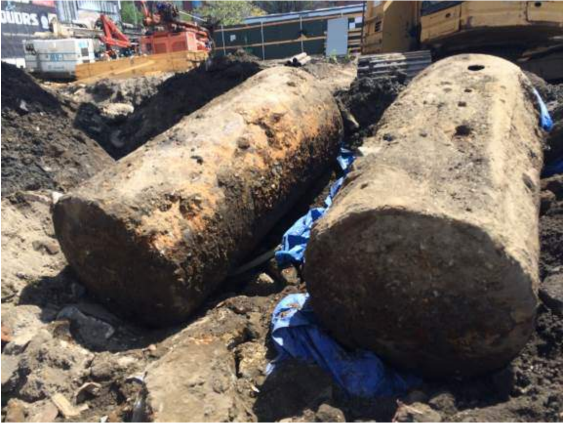
Photograph 9: View of the removed USTs (UST-12 and UST-13).
