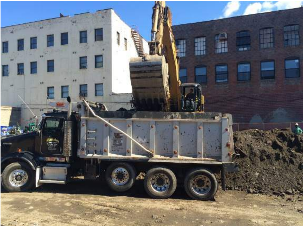
Photograph 10: View of the contractor directly loading material for off-site disposal to Clean Earth of Carteret, in Carteret, New Jersey.
