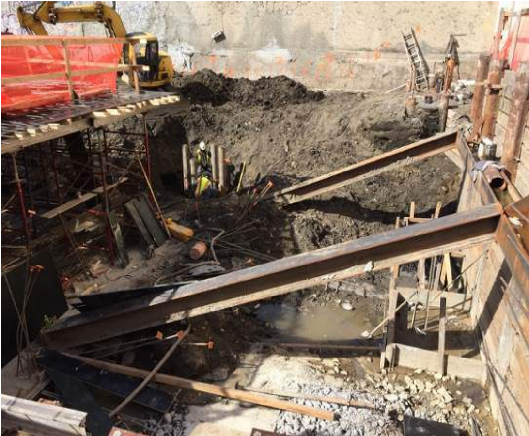
Photograph 102: View of the contractor welding the piles, facing southwest.
