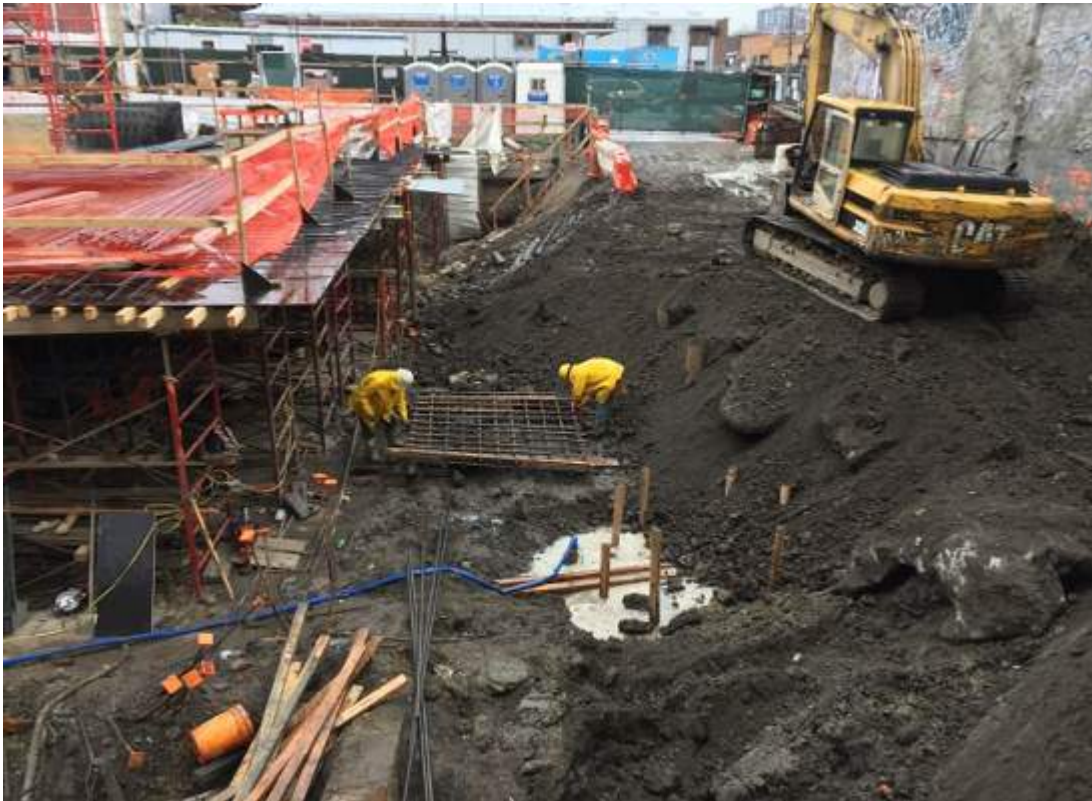
Photograph 104: View of the contractor dewatering the pile cap area, facing southwest.
