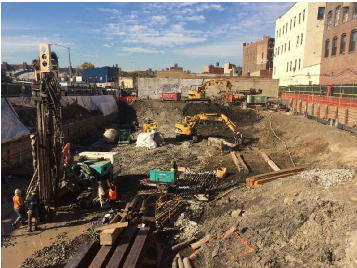
Photograph 42: View of the site progression, facing northwest.
