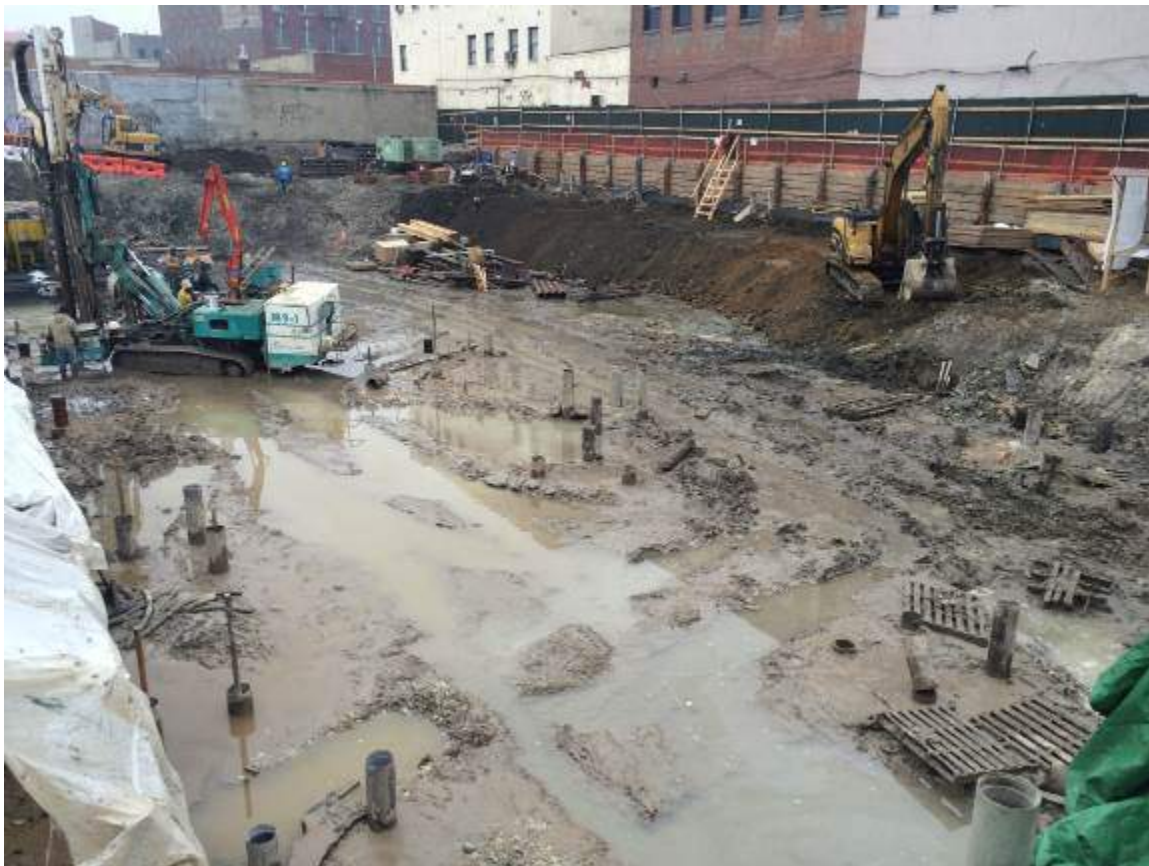
Photograph 48: View of the site progression, facing north.
