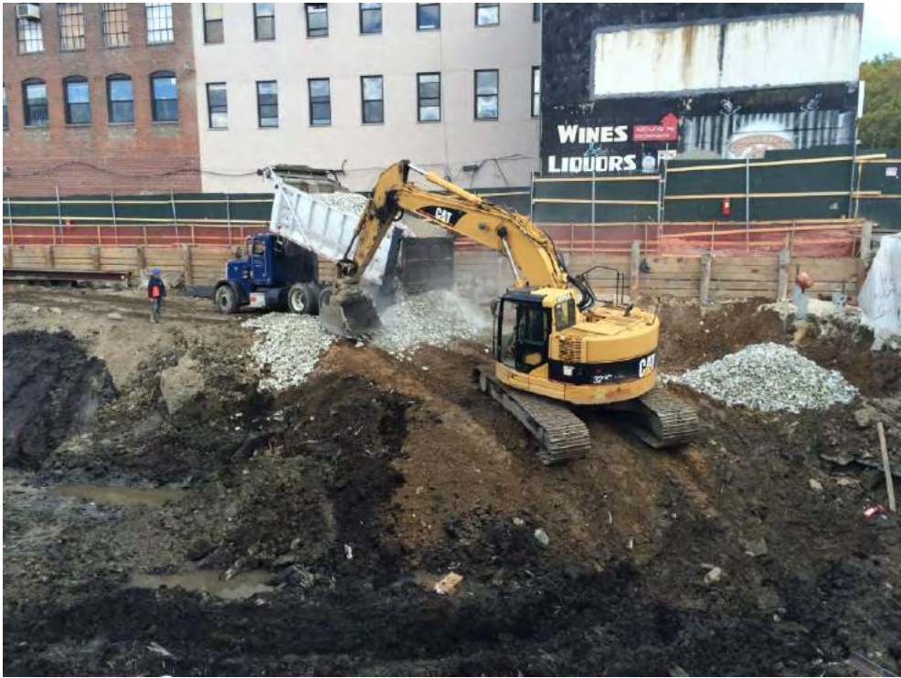
Photo 5 – View of the contractor unloading the stone.
