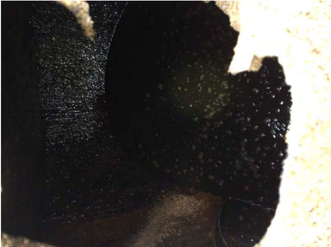
Photo 6 – Interior view of UST-14.
