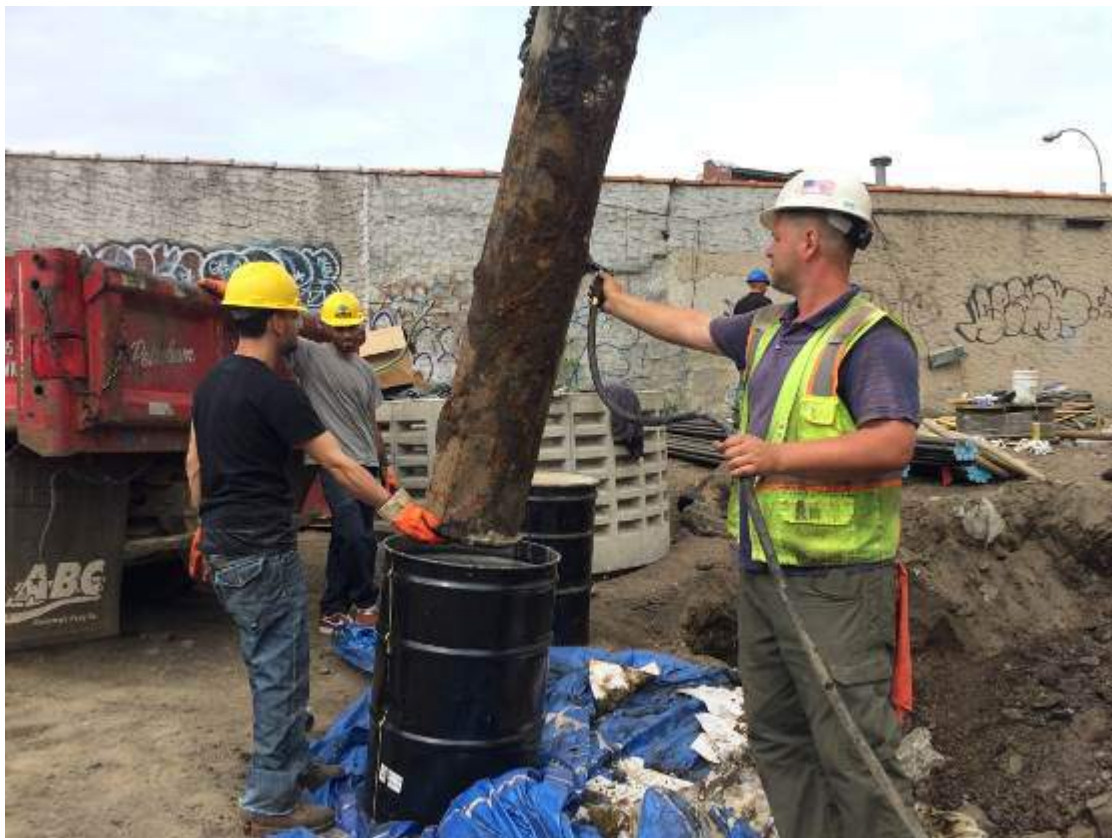
Photograph 30: View of the hydraulic fluids of Lift-2 being emptied into a 55-gallon drum.
