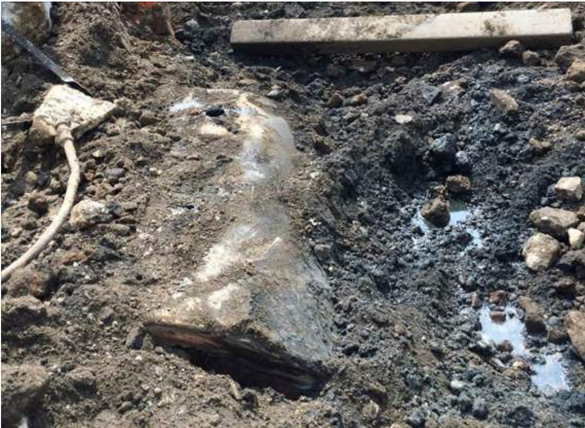
Photograph 12: View of UST-15 discovered north of UST-14.
